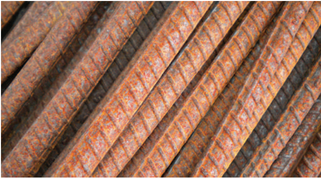
Figure 4 – Overall view of #3 bars left exposed outdoors for 20 months.
